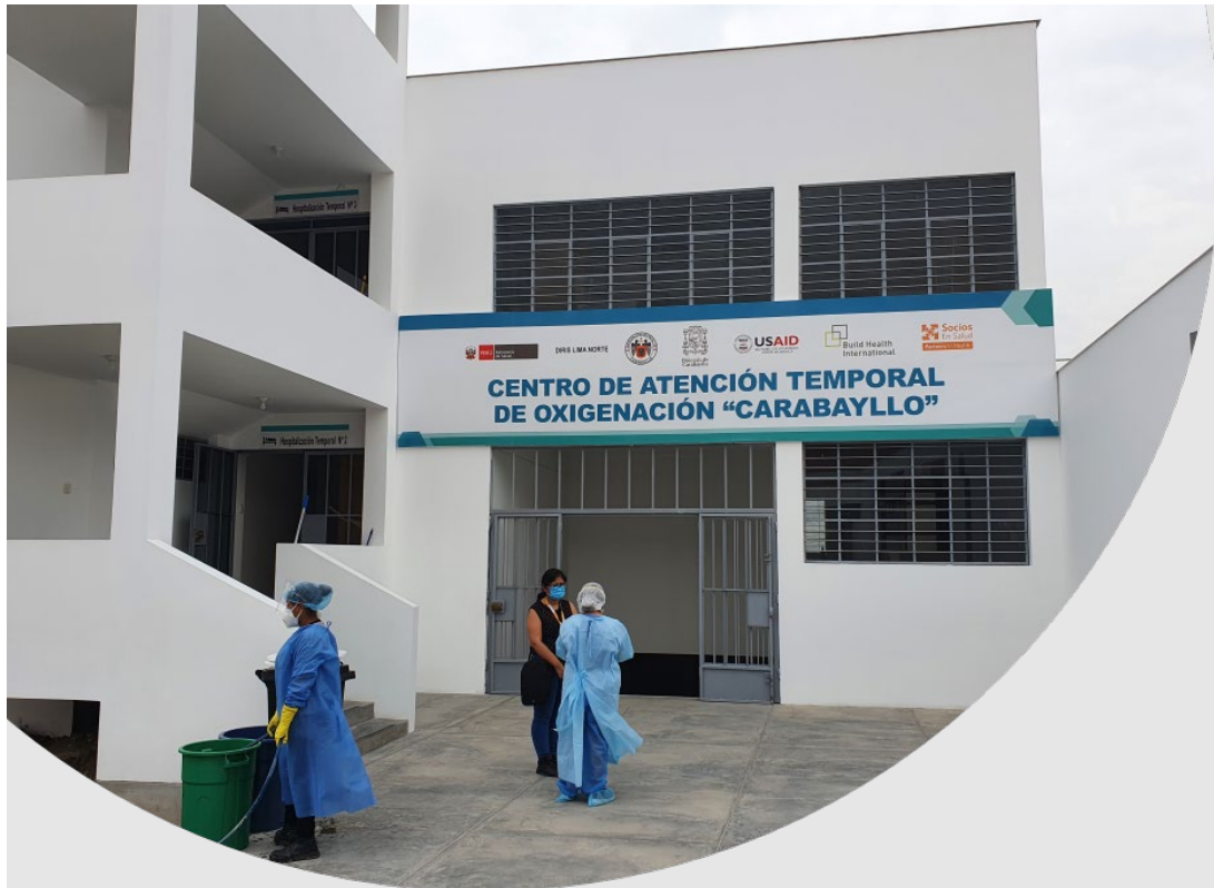
Figure 19. Installing TOC Carabayllo
