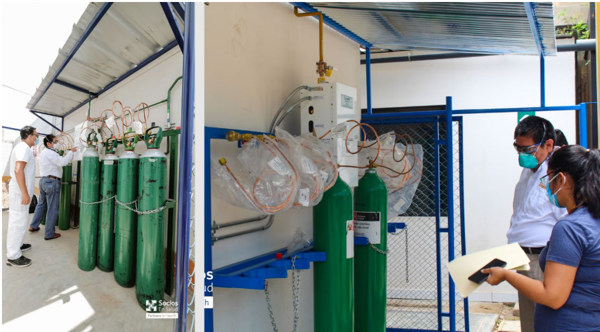
Figure 21. Installation of Oxygen Manifold Panels, Trujillo
