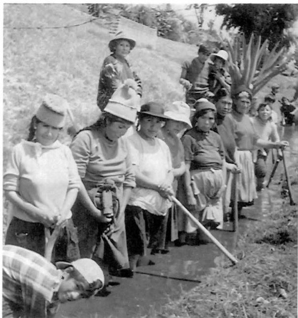
One of 834 small high-impact, community-level projects financed by USAID-Peru's Special Development Activities Program, completion and rehabilitation of Pilcomayo's potable water system by residents affected approximately 2,000 families.
